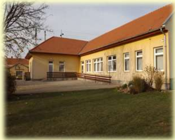
the building of the kindergarten /Felsődobsza/
